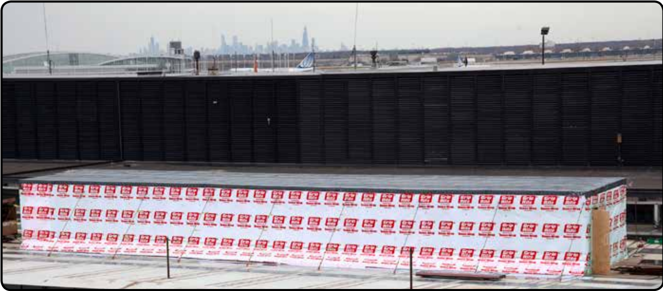
Grip-Rite Weather Resistive Barrier used at O'Hare International Airport
